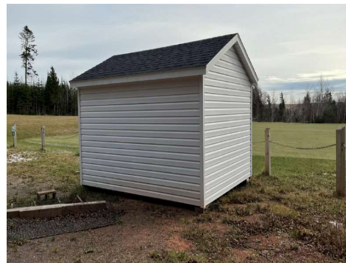
Figure 6 – Rear of Shed
